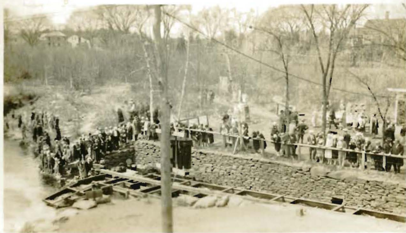
THE NEW BRIDGE
