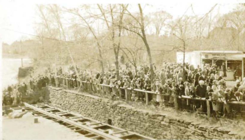
THE NEW BRIDGE
